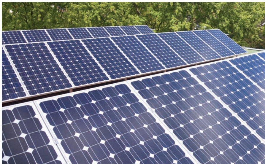
PV modules installed in rows and tilted up require careful placement to avoid one row shading the next.
