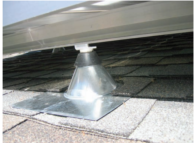
The modules in this array are about six inches off the roof, allowing adequate ventilation to keep them as cool as possible.
