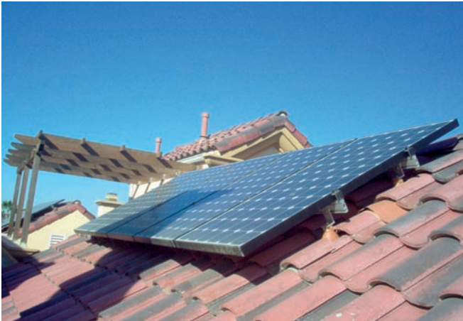
Overhangs, second stories, trees, vents, chimneys, etc. can affect the output of a PV system. Some potential shadings are hard to detect in advance without careful siting efforts.
