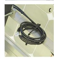
Almost all modern PV modules come with prewired, multicontact (MC) connectors. These connectors simply plug together, allowing fast installation and a low-resistance, weather-tight connection. MC connectors should be firmly pushed together and given about a quarter turn to make sure the seal is tight. Your system design will determine how many modules will be wired in series, and how many series strings your array will have. (See my article on wiring configurations for a PV array in *HP87*.)
