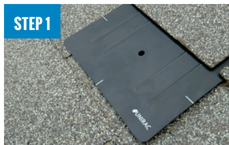
STEP 1 INSTALL FLASHKIT PRO FLASHING
