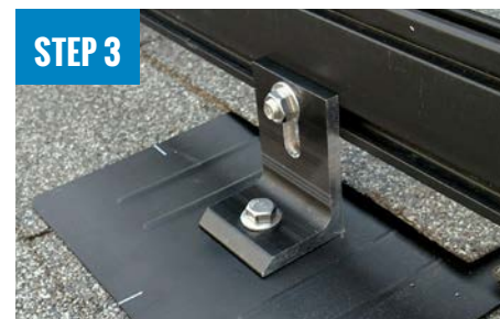
STEP 3 ATTACH L-FOOT TO RAIL
