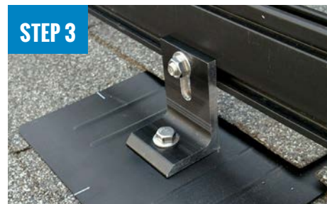
ATTACH L-FOOT TO RAIL
