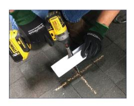
As the lag screw is being driven into the roof, watch rubber gasket on underside of sealing washer for compression. Stop driving the lag screw when the gasket becomes visible around the edge of the washer.
