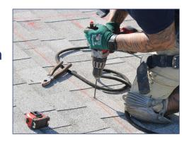
Remove any dirt or debris from roof surface and properly seal any missed pilot holes with a flashing card before SpeedSeal™ Foot is installed.
