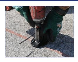
6 As the lag screw is being driven into the roof, watch rubber gasket on underside of sealing washer for compression. Stop driving the lag screw when the gasket becomes visible around the edge of the washer
