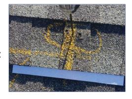
Turn SpeedSeal™ Foot over and apply roof sealant, filling the cavity formed by the sealant ring.
