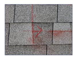
Using locations drawn on roof during system layout, drill a 3/16" pilot hole into roof framing member.
