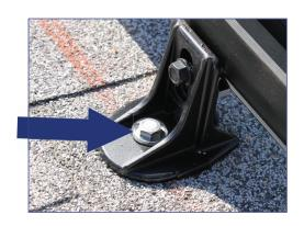
As SpeedSeal™ Foot is tightened to the roof sealant will ooze from the lower cavity of the L Foot as an indicator of proper sealing. If no sealant is seen, remove SpeedSeal™ Foot from roof and add more sealant before reinstalling.
