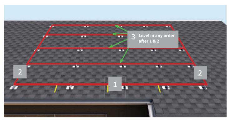
To level top sliders to the same height in the first row, run a string line between the first and last mounts in the first row. After aligning the first row horizontally, follow the same string alignment process vertically on far right and far left columns. Then align each remaining row of the array (in any order).
