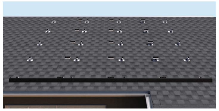
Only the front row needs to be aligned and locked down in order to assure a straight and secure skirt and array. The clamps in the rest of the rows will self align as you install the modules and do not need to be aligned or locked into the base mounts. For optional skirt attachment method see the full *Quick Rack Installation Manual*.
