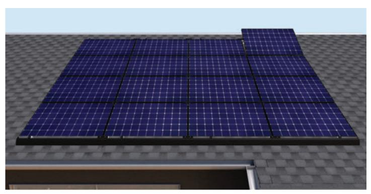
The upper row of clamps should remain loose to accept the next row of modules. Complete wire management for the first row and then continue installing modules for all rows, tightening the lower row of clamps and completing wire management for each row as it is installed. Tuck the wires inside the module frame with wire clips on each side of the connectors. See the full *Quick Rack Installation Manual* for more information on wire management configurations and wire clip recommendations.
