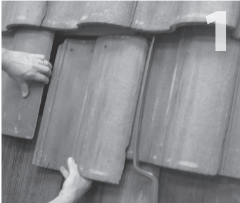
Remove tile at selected location of mount.
