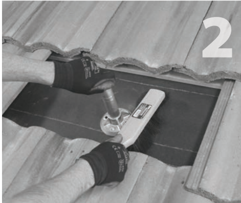
Clean away dust and debris around QBase.
