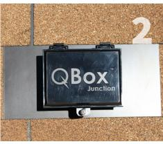
Slide the QBox flashing up underneath the second course of shingles, so that the bottom edge of the flashing does not overhang the front edge of the shingle and the top edge extends up into the third course of shingles.
