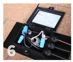
Push Wires Into Box: Push wires down into the box and away from the lid. Lid should close freely without wire interference. Failure to do so will prevent proper rainproofing of the enclosure, voiding the warranty and possibly leading to a short. Secure the lid per step 12 in section IV.
