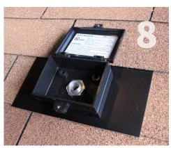
Reinstall Flashing: Reinstall the QBox assembly such that the conduit fitting in the center of the box aligns with the hole you created in step 4.
