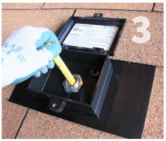
Mark Conduit Location: If not using attic conduit exit, complete only step 6-8 and 11-12. Otherwise, remove the conduit cap and blank and set aside. mark the location to drill the conduit pass-through with a lumber crayon or other marking device.
