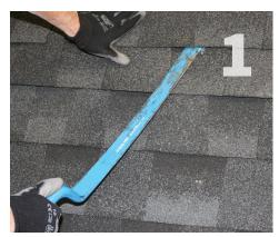
Remove Nails: Use roofing bar to break seals between 1st and 2nd and 3rd shingle courses. Be sure to remove any obstructing nails to allow correct placement of the QBox.
