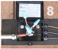
Connect Wires: Pull min 6" of transition wiring into the QBox, label all wires, and strip sheathing from the end of all wires per the instructions of the manufacturer of the connectors being used. Follow step 6 to complete the installation.
