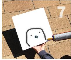
Optional Caulk: Apply an upside down U-shaped bead of sealant to the underside of the flashing before insertion. Do not use excessive sealant.
