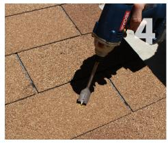
Drill Conduit Hole: Remove QBox flashing and drill 1" hole at location marked in Step 3. Use either a spade bit or hole saw. Avoid all electrical components on underside of deck in the attic.
