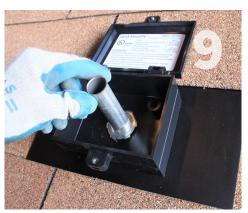
Install Conduit: Install the supplied conduit nipple through the QBox and the roof with the flared end facing up.
