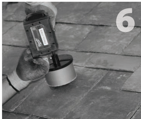
Using a 4" diameter diamond hole saw and the pilot hole drilled in step 3, drill through the existing slate.
