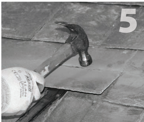
To remove the slate below the score, slightly lift the lower portion of slate with a slate ripper, then gently but firmly tap the top piece with a hammer. The lower piece should break off cleanly.
