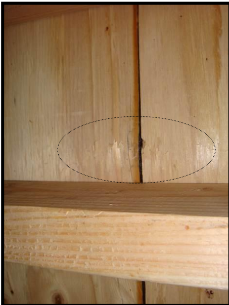
Figure 4a. Buckled Plywood Shear Perpendicular to Rafter
