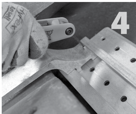
4 Slide hook into desired position within valley of the tile. The hook must not overhang the side edges of the base plate. Tighten set screw (item 4) with hex key.
