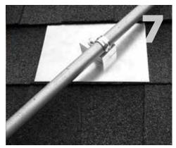
Insert lag through hole in block, and position clamp over conduit. Using drill with 7/16" socket, drive lag until block is tight.
