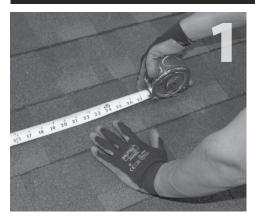
Choose placement of conduit mounts along path of conduit. Select location over center of rafter.
