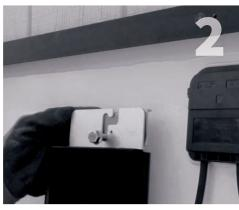
With the cap screw threaded into the bracket, slide the cap screw into the slot on the module level electronic mounting bracket with the bracket behind the module level electronic mounting bracket.
