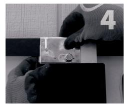
Place the frame clamp over the edge of the module frame, and in front of the module level electronic mounting bracket. Slide the assembly up and to the left to engage cap screw into frame clamp slot.
