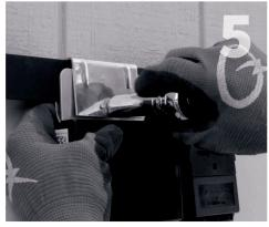
Tighten the cap screw with a half-inch socket and torque wrench to a torque of 15 foot-pounds.
