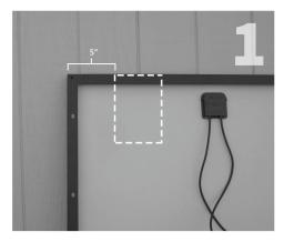
In a standard landscape or portrait array, the Accessory Frame Bracket should be installed at least 5 inches from the edge of the module and at least 1 inch in from the edge of the module junction box.
