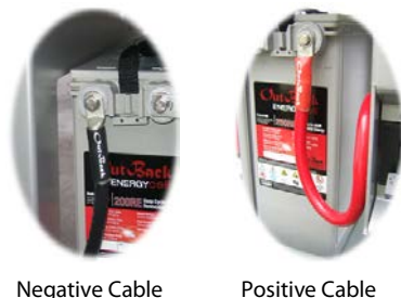
Figure 5 Battery Interconnect Bars and Hardware
