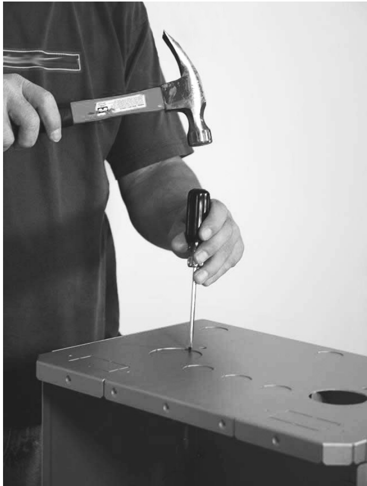
Figure 6: Removing chassis side knockouts
