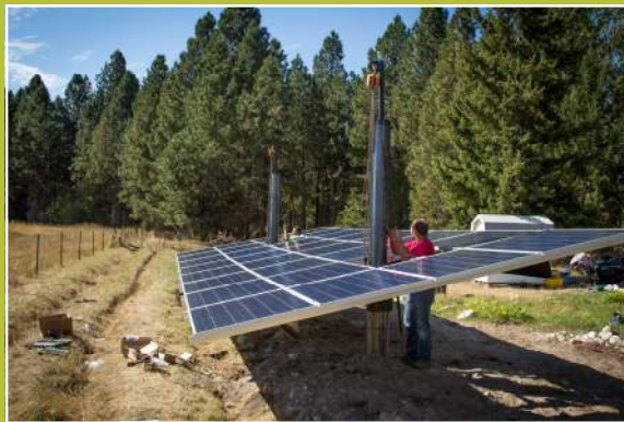
HOIST FROM THE GROUND
