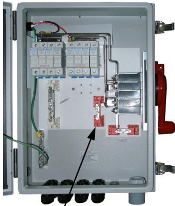
Step 4: Reinstall Positive block
