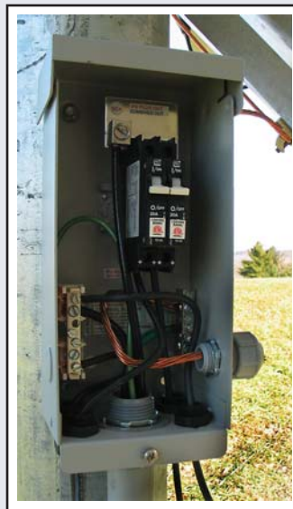
Installation photo courtesy of APRS World
