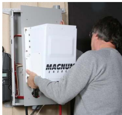
Figure 10, Ensuring door is in all three hinge openings and moves freely
