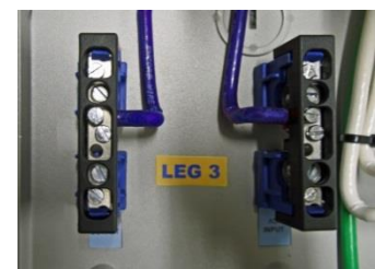
Completed. Red wires replaced with blue and "LEG 2" Sticker replaced
