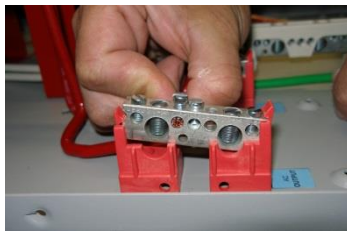
Finish removing the terminal block
