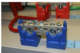
Replace the Busbar and press into place
