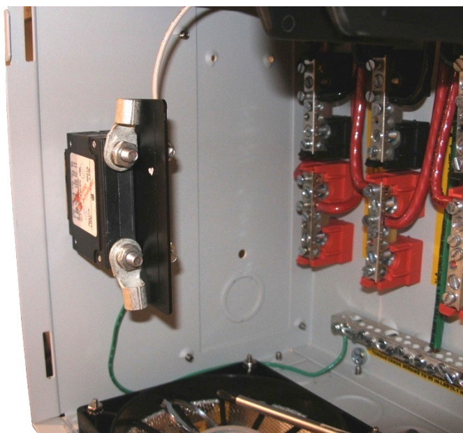
80 amp panel mount DC-GFP ready for the high current wires.
