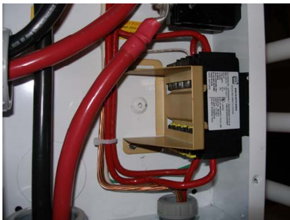
Din Rail mounted breakers
