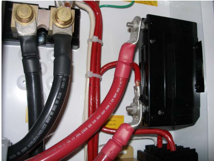
Battery Positive connections and shunt wiring
