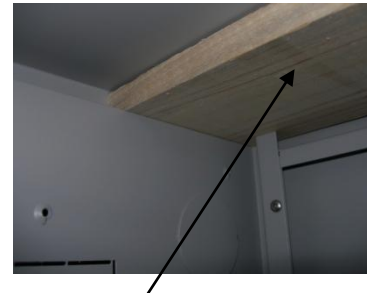
3/4" Piece of wood added as support
