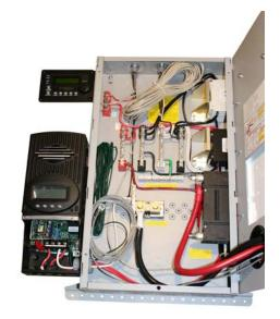
Magnum all wired up and tested with lightning arrestors, charge control disconnects, charge controller and remote display ready for transport to the job site. A DC-GFP and battery status monitor could also have been added to this assembly.
