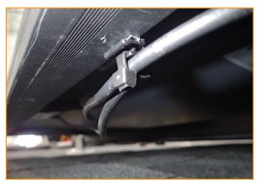
Install wires inside Aire Rail and wrap the Cable Tie around the rail to secure the wires in place. Cut off any remaining cable tie after installation. Modules must cover all wires after installation. There shall be no visibly exposed wires after installation of modules.
