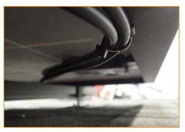
When running wires north/south or east/west under a module, attach Edge Clip to module frame flange and use Cable Tie to secure wires to module frame, or use Cable Ties to secure wires to rail. Cut off any remaining cable tie after installation. All wires must remain underneath the module after installation. There shall be no visibly exposed wires after installation of modules.
