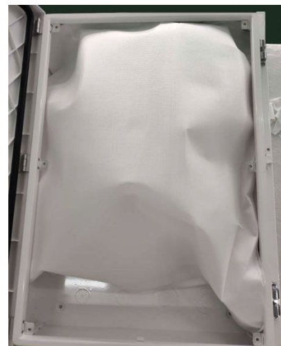
Internal components protection
