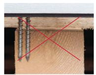
Rafter might split – fasteners are mounted extremely close to the edge.
