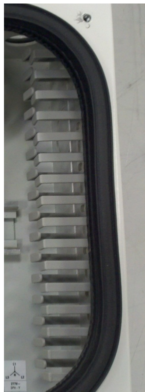
Front switch – cable guides
